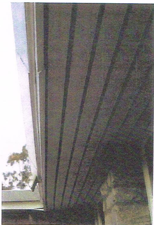
EXTERIOR NW SIDE
