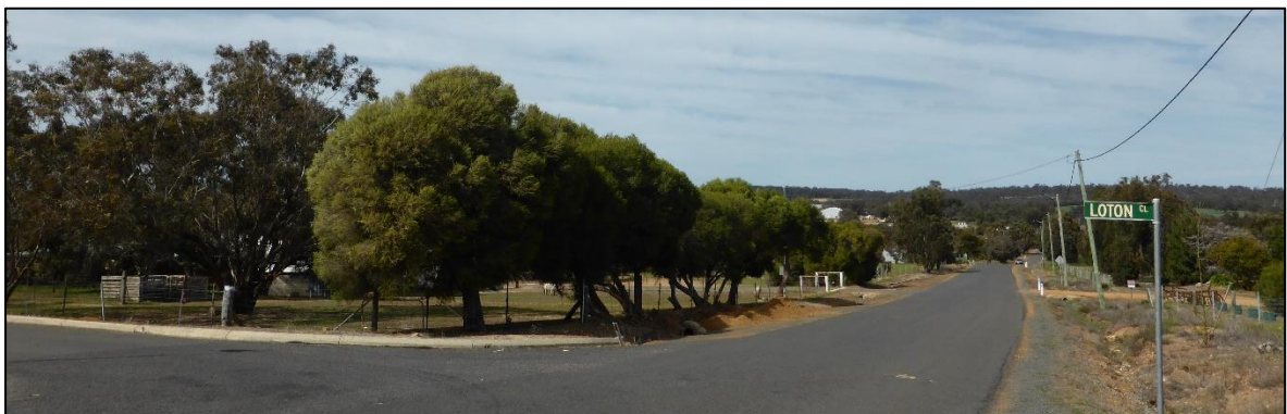
(Work yet to commence at Loton Close on Independent Living Units – September 2015)
