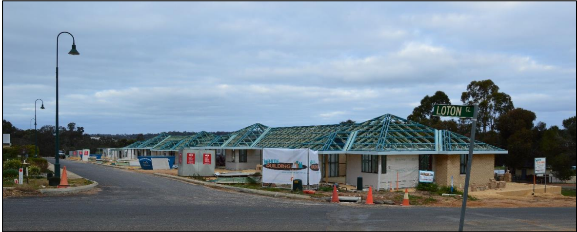
(Construction in progress of Independent Living Units – July 2016)
