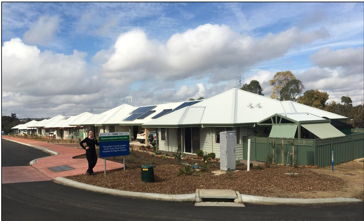
(Completed Independent Living Units with Landscaping – June 2017)
