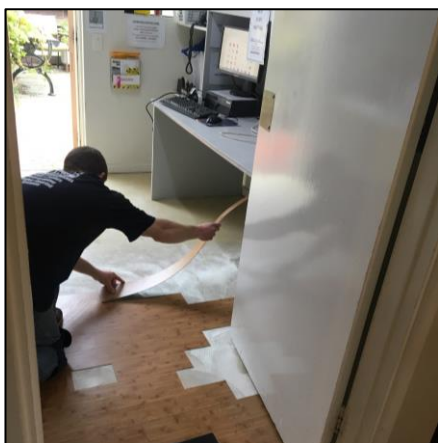
(Springhaven Lodge – Stage 2. Left – Vinyl flooring going down. Right – Hairdressing facilities going in.)
