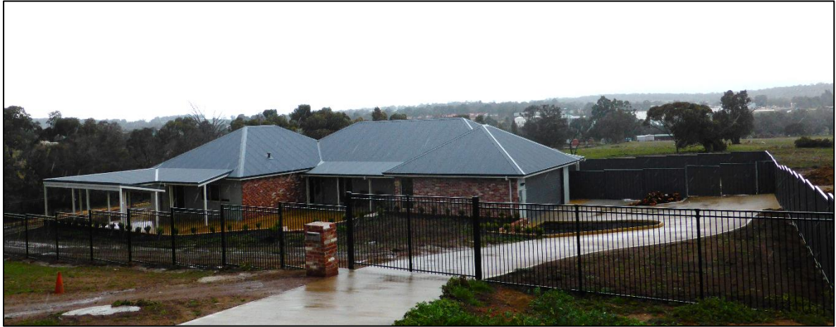
(Completed Executive Residence – June 2017)
