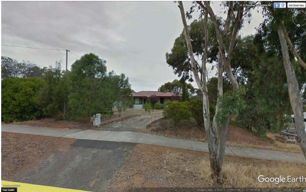
Street view image showing front of property from Kojonup-Katanning Road and existing driveway and dwelling (Source: Google Earth Pro)
