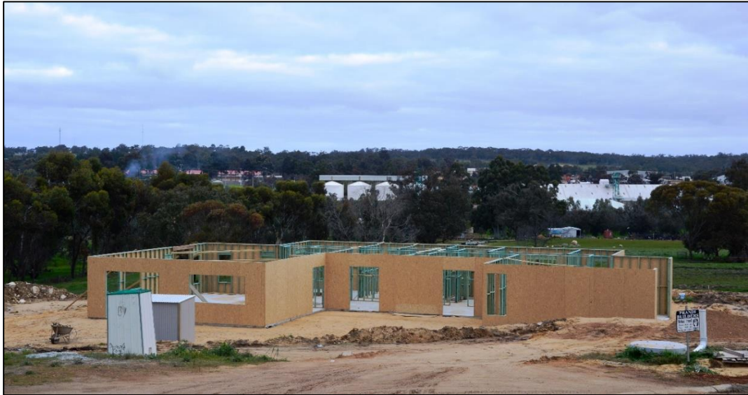
(Work in Progress – 12 July 2016)
