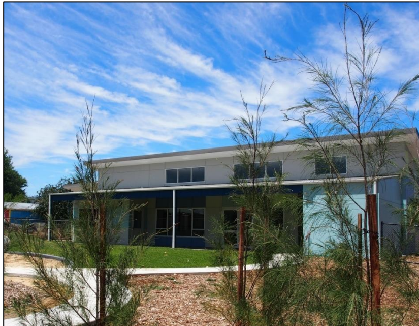
(Source: H + H Architects – Completed – February 2016)
