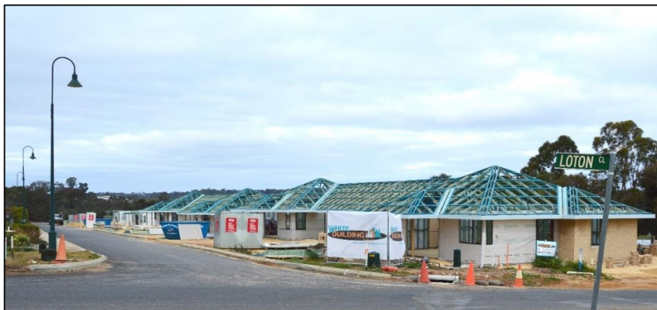
(Work in Progress – 12 July 2016)
