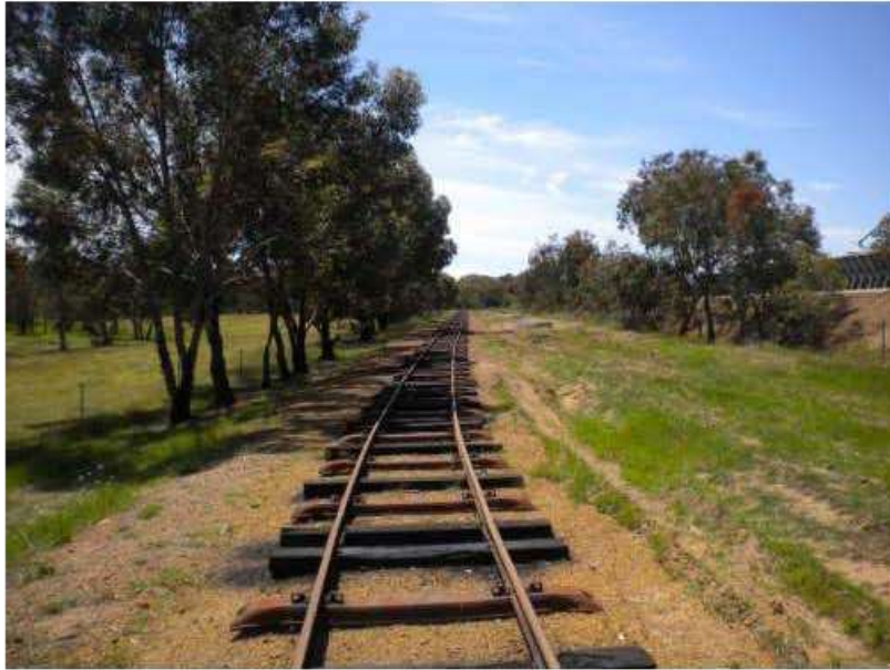
View looking back to Pensioner Road
