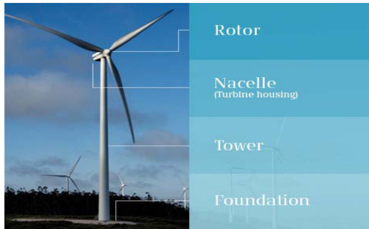
Figure 6: Anatomy of a Wind Turbine Generator
