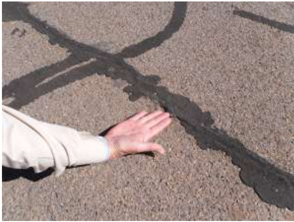
The Two Eastern end Netball Courts are a High Trip Risk and not fit for safe use
