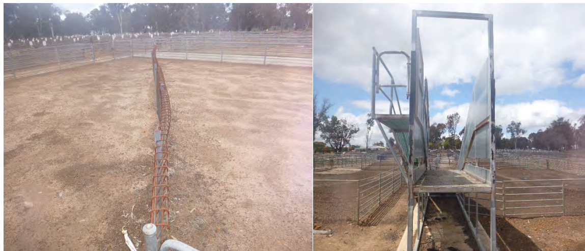
Photo 3 Weldmesh panels in situ Kojonup Saleyard and 4 showing lack of bump rubbers.
