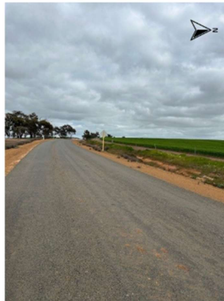
Jingalup Road - Proposed Site Entrance (facing West)
