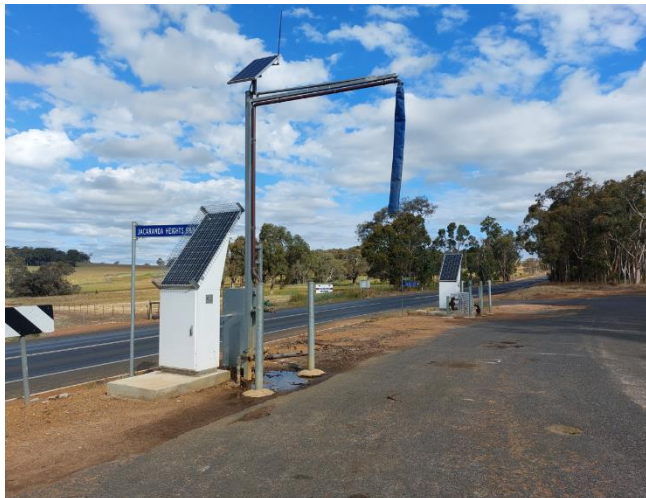
Standpipe situated next to Albany Hwy south of Stock Road. Overhead standpipe – scheme water (fees payable)
