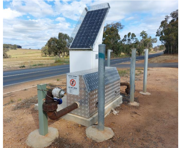
Non-potable coupling water supply
