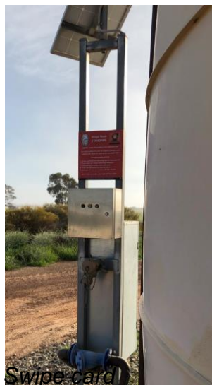
Tank, electric swipe card and pump for bore
