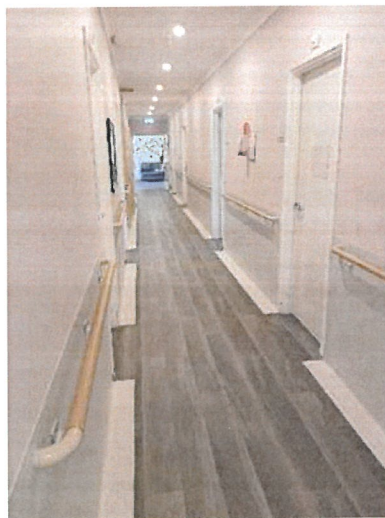
Springhaven - New Railing
