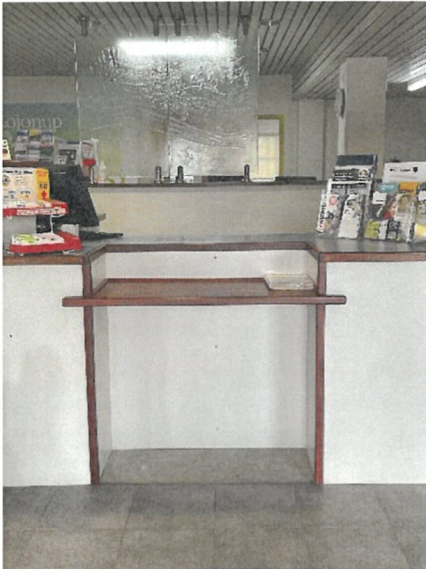
Modifications to Administration Building Front Counter to provide for easier access
