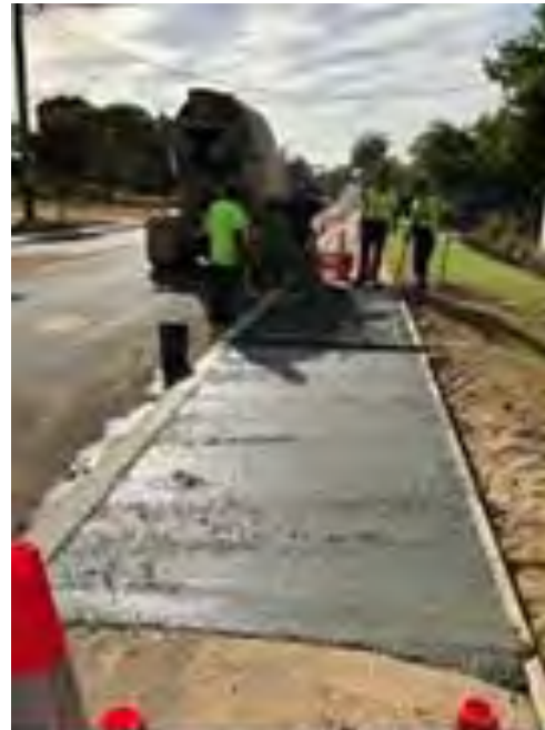
Kerb laying - Spring Street
