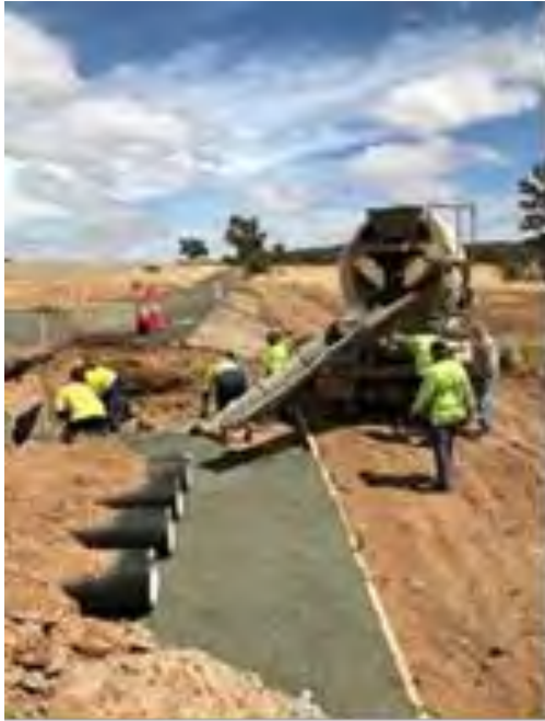
Installation of a new culvert Riverdale Road
