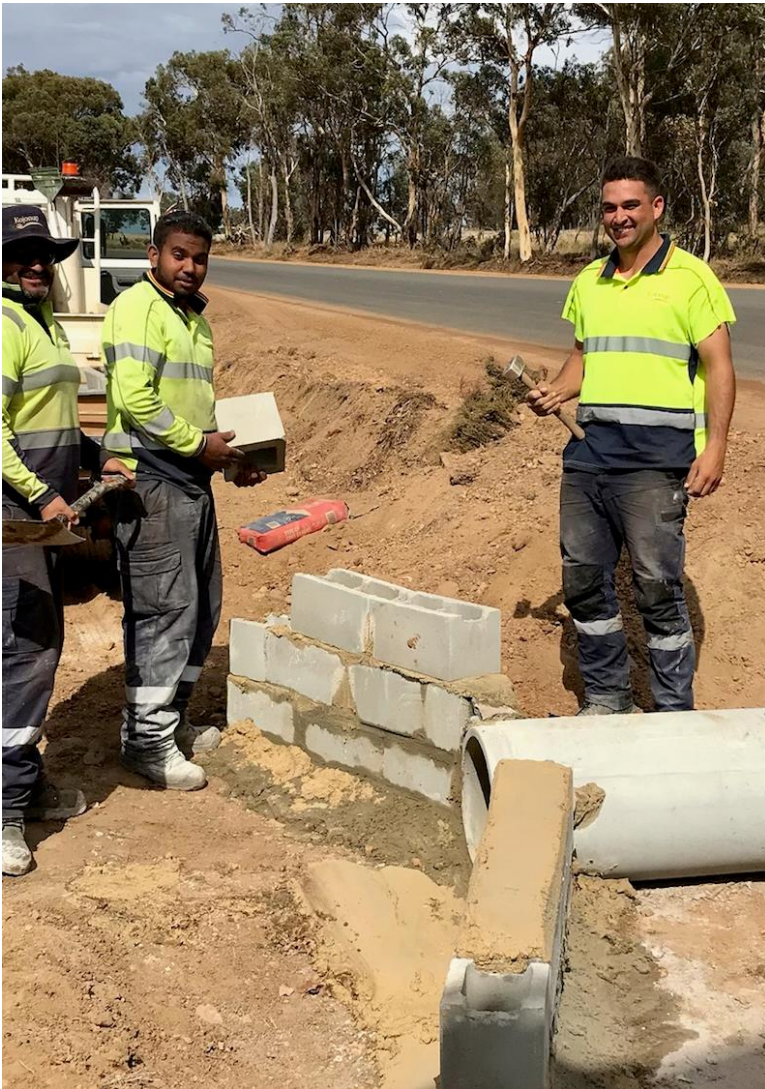
Depot crew extending a culvert and building headwalls on Shamrock Road widening project.
