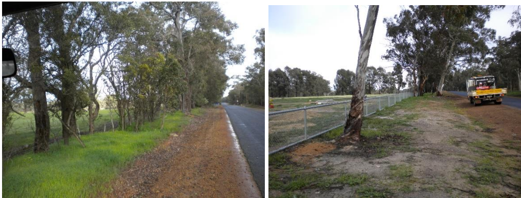
Tunney Road before spraying 9 October 2018
