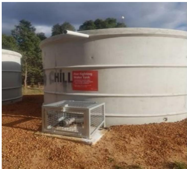
Example Strategic 47,000 Litre Concrete Tank & Protected Fittings
