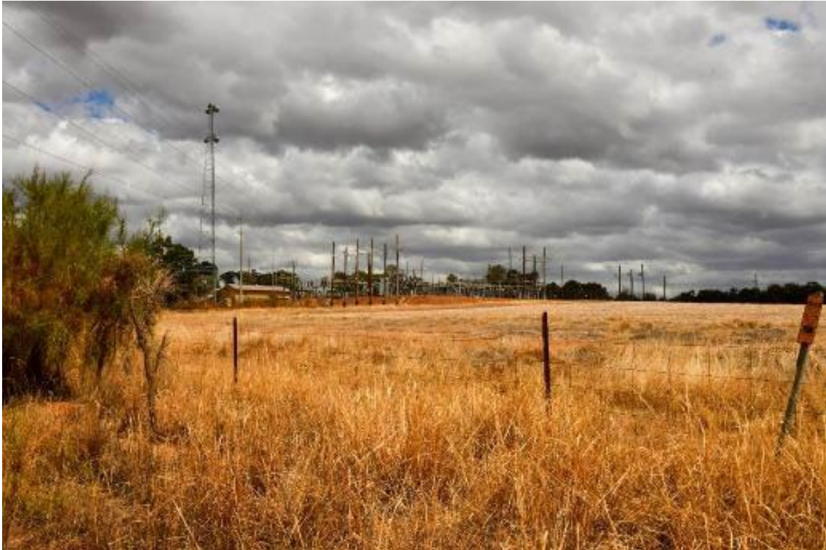
Figure 11: Typical View of LCU3 showing Substation and Mast Tower (located to the left side of the photograph)
